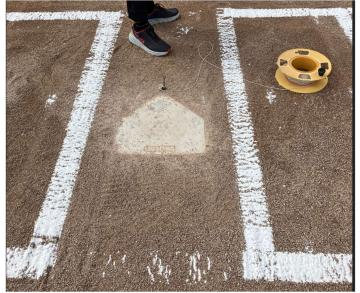
• Run the stringline all the way to the edge of the infield and ensure the string is straight with the outside edge of the base (or baseline survey pin)
